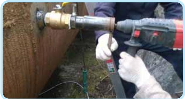
Insertion Transducer Installation
